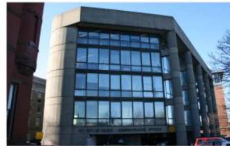
COUNTY OF ESSEX – ADMINISTRATIVE OFFICES
